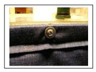
I also found that the product needs to be supported at both ends; otherwise, the small brass screws begin to pull out of the pine components as shown below.
